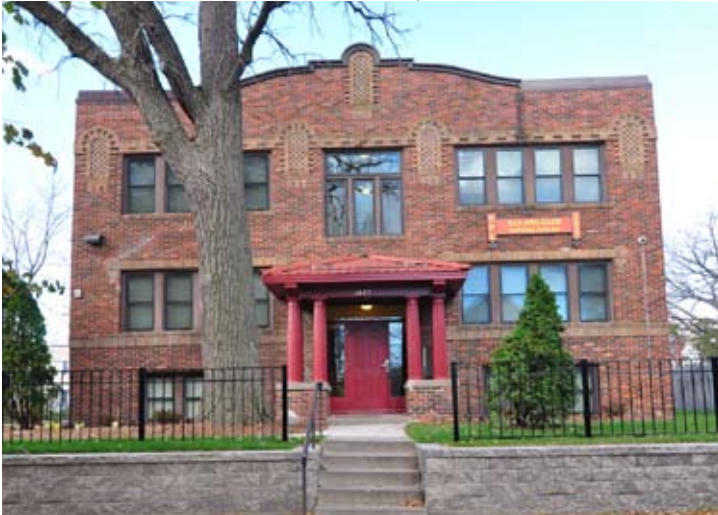
NEAR NORTH REHABS, MINNEAPOLIS
