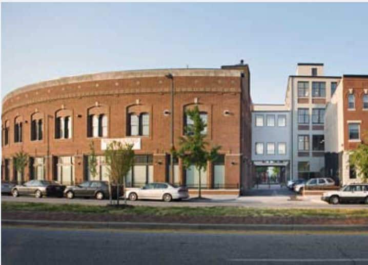
PRINTERS' SQUARE APARTMENTS, BALTIMORE
