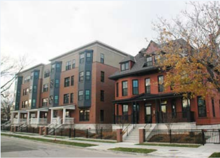
ALLIANCE ADDITION, MINNEAPOLIS
