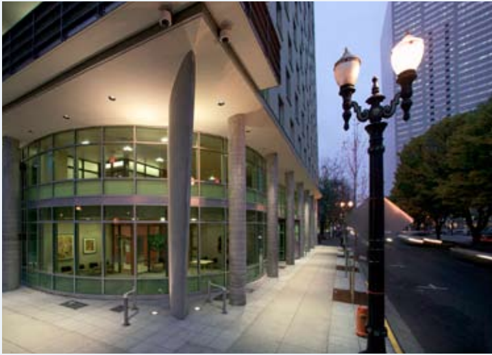
RICHARD L. HARRIS BUILDING, PORTLAND
