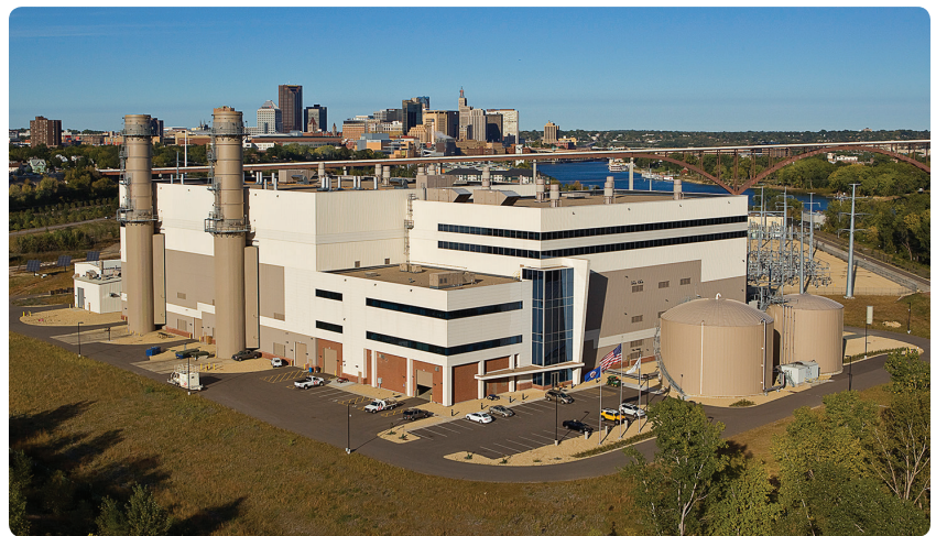
Converted for natural gas production, the Xcel Energy High Bridge Generating System in Saint Paul came on line in May 2008.
